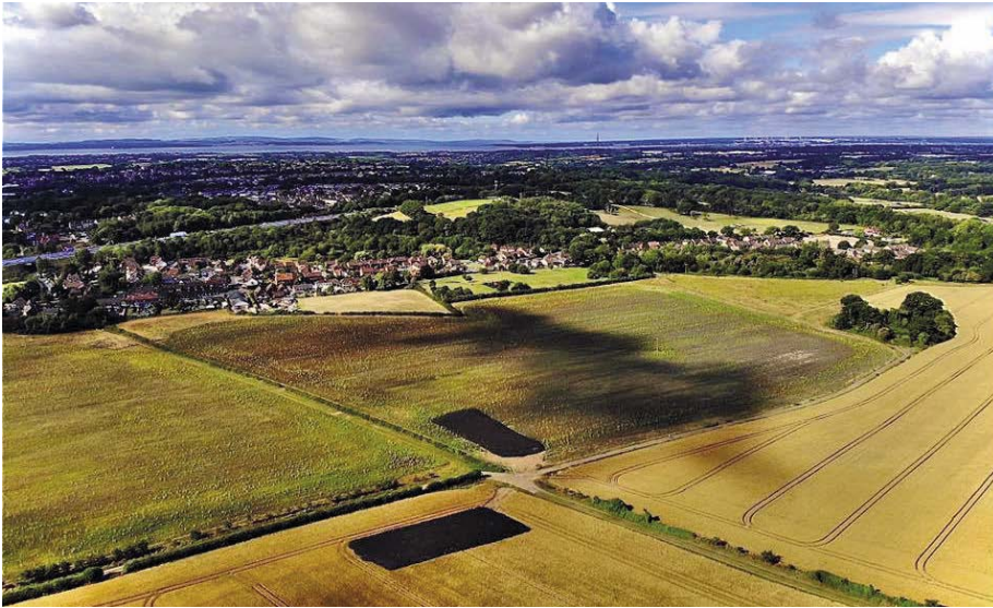
Fields north of Funtley where Welborne Garden Village will be built (Adrian Saunders)
